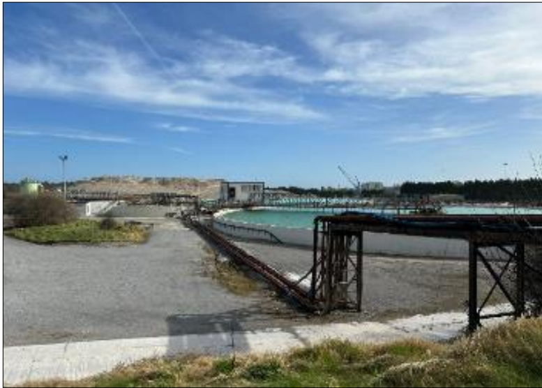
Plate 15.23: Settlement ponds and, in the background, the large stockpile area
