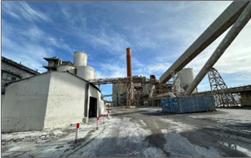
Plate 15.15: View looking east within the area of the magnesia and magnesium hydroxide facility
