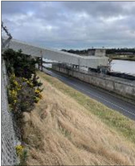
Plate 15.21: View towards the loading wharf/pier
