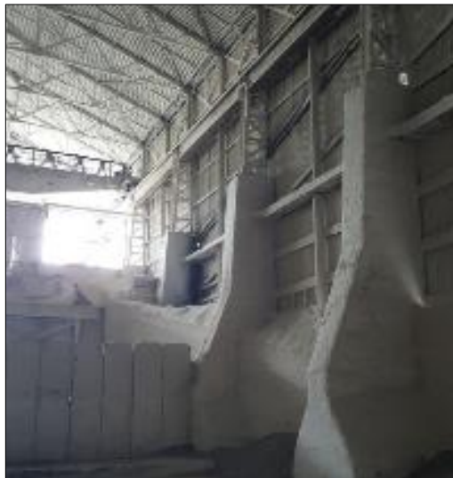
Plate 15.14: Interior of the crane store structure (showing detail of the integrated gantry). This end of the structure is to be retained
