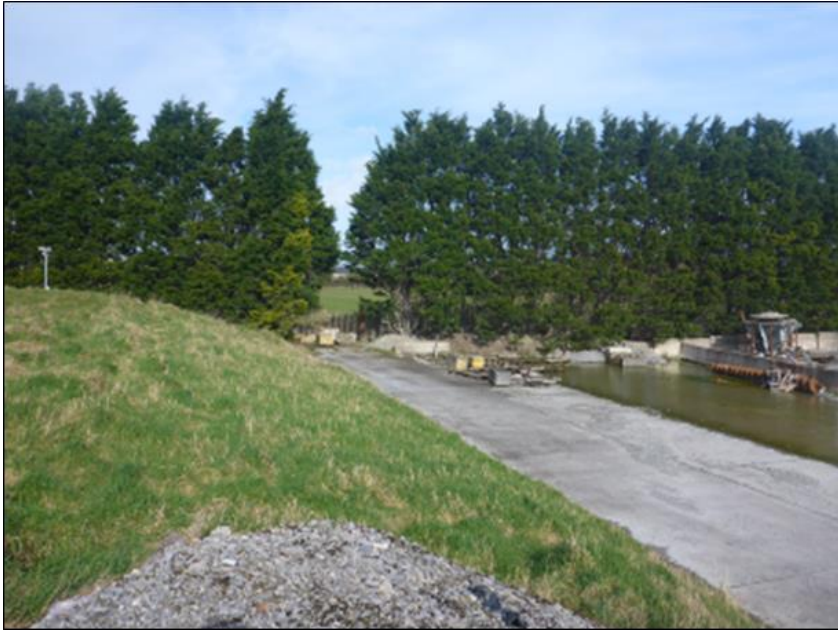
Plate 15.7: View from the stockpile, looking north to the secondary entrance to the site. Note the difference in elevation of the landscaped to the fields to the north
