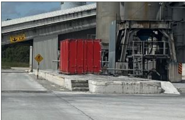
Plate 15.22: Detail of the concrete railway platform
