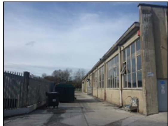
Plate 15.4: Side (southern) elevation of the workshop
