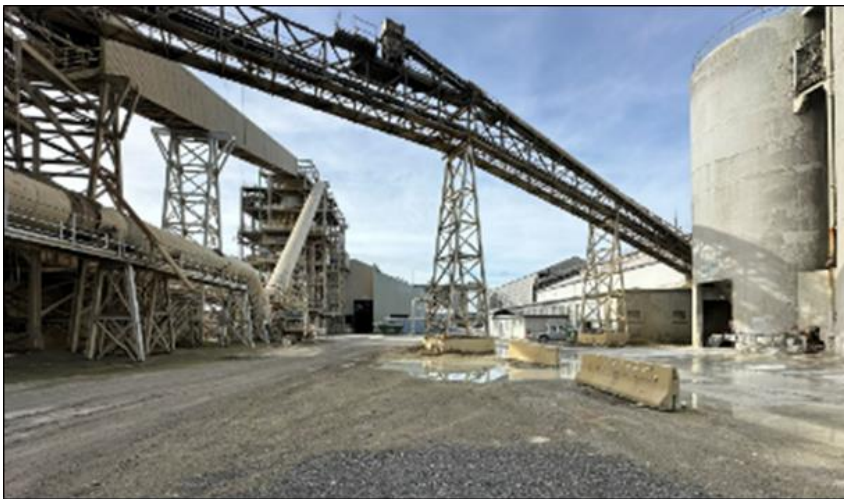
Plate 15.16: View looking west within the area of the magnesia and magnesium hydroxide facility
