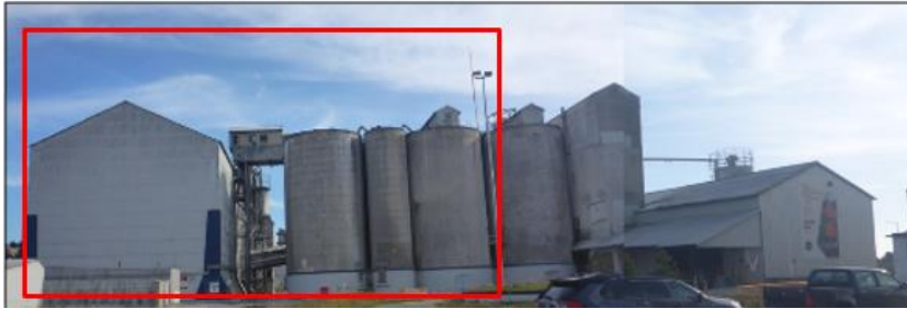
Plate 15.12: View looking east of the crane store (CH3), silos (CH2) and, rotary kiln building at the western end of the site (Stitched image). The highlighted structures will be retained/partially retained in the Proposed Development
