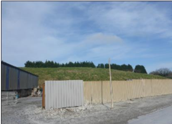
Plate 15.8: View towards the northeast of the stockpile in the northern central area of the site
