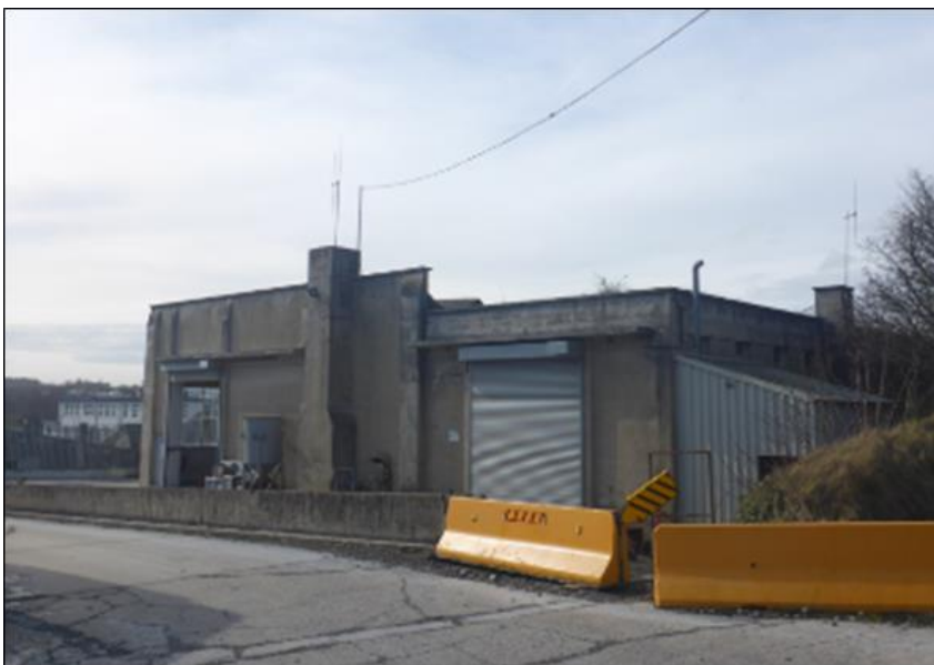
Plate 15.5: View to the southeast of the front façade and side elevation (northern) of the workshop
