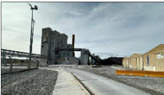
Plate 15.17: View looking east of the magnesia and magnesium hydroxide facility and shaft kiln brick shed on the left-hand side
