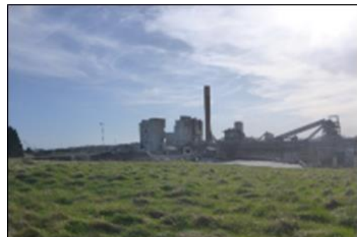
Plate 15.18: View looking south of the buildings on the site from Stockpile 1.
