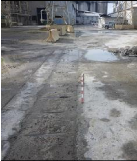
Plate 15.19: Remnant of the train track within the site cut by a drain
