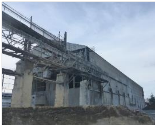
Plate 15.13: View towards the southwest of the crane store structure
