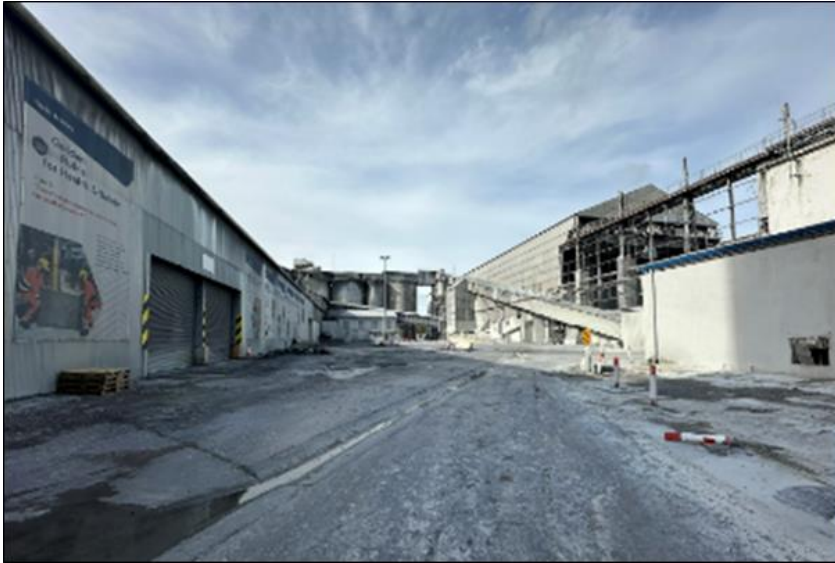
Plate 15.10: View west towards the rear second bank of silos from the centre of the production facility area and rotary kiln building on the left-hand side.
