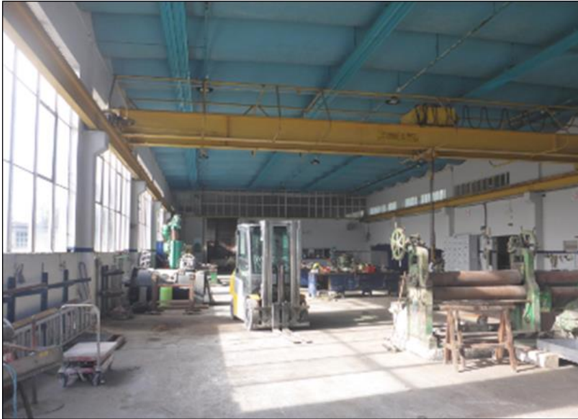
Plate 15.6: Interior of the workshop showing roof detail and internal gantry crane
