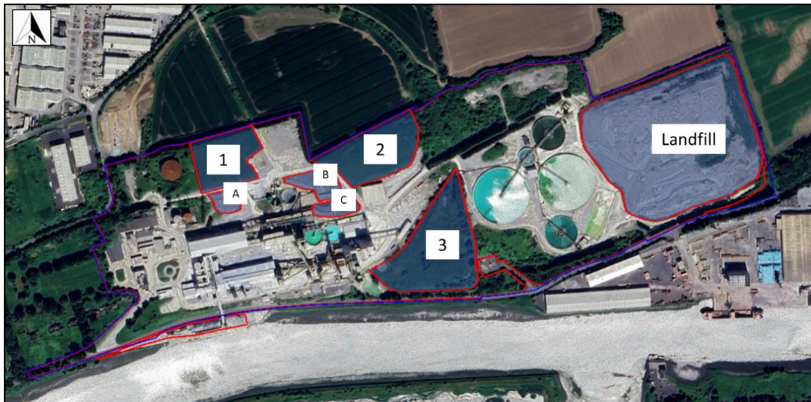
Figure 14.1: Aerial photograph showing location of the on-site landfill and stockpiles 1, 2 & 3 (Spoil Heaps A, B & C as described in Chapter 7 Soils Geology and Hydrogeology as shown)
